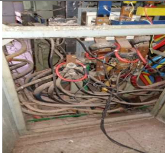
Main cable termination in LT panels
