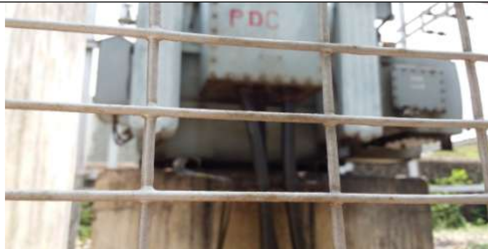
Transformer Oil Leakage
