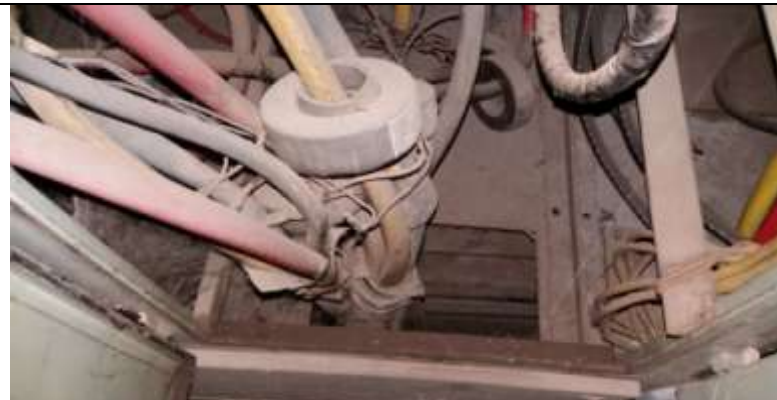
Main cable termination in LT panels
